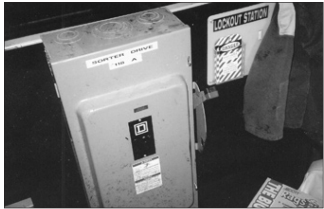
Fig. 2: Lumber mill conveyor lockout/tagout with tags available.
